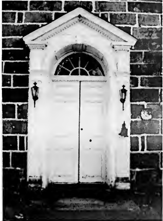
Figure 19 Front Entrance of the South Wing of the Main House, 2001
